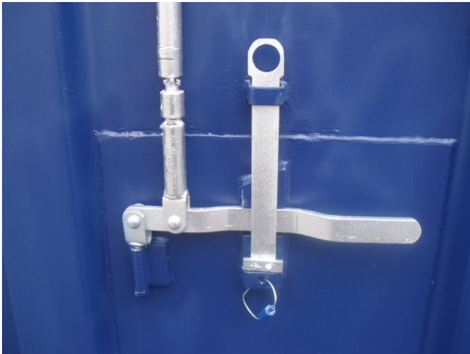
Roof Locking Device (Total Six Sets At Both Sides)
